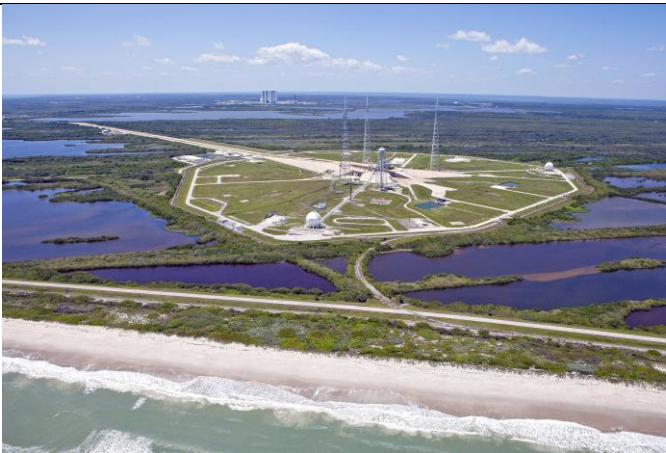
The refurbished Launch Complex 39B at Kennedy Space Center, which is on the ocean and surrounded by marshland, in 2013
